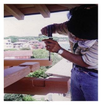
Figure 1. Carpenter cutting joinery
